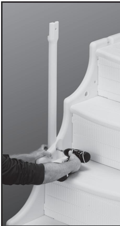
**#1:** Attach one of the four rail posts by aligning the two holes in the bottom (round end) with the two holes in the lower post location on the side panel. Push the two 2-1/2" bolts through the holes from the inside of step to the outside. Secure with two 1/4" x 20 hex nuts.
