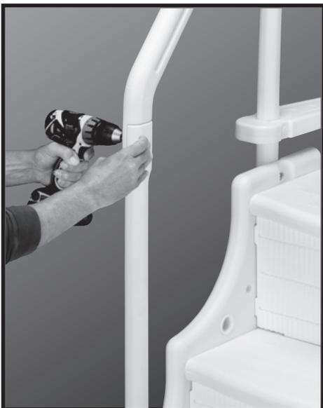
**#5:** Match the indents on one of the handrails with the indents on the rail posts and attach the handrail using two 2-1/2" bolts and two 1/4" x 20 hex nuts.
