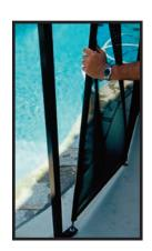
A. Once fence panels have been installed and tension applied, hang gate by attaching hinges to frame with the self-tapping screws supplied.
